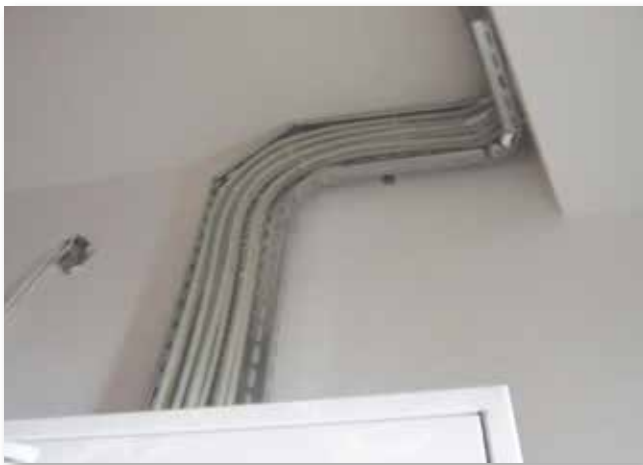
Cables are installed into a single duct in buildings.
