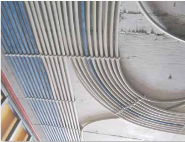
Cables are installed by being pushed through the ducts.
