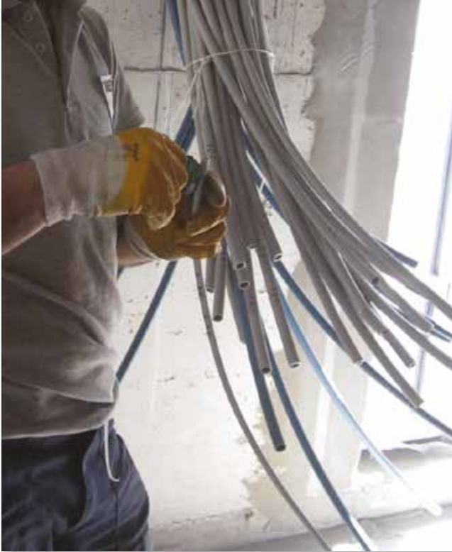
An operator stripping cables during installation.
