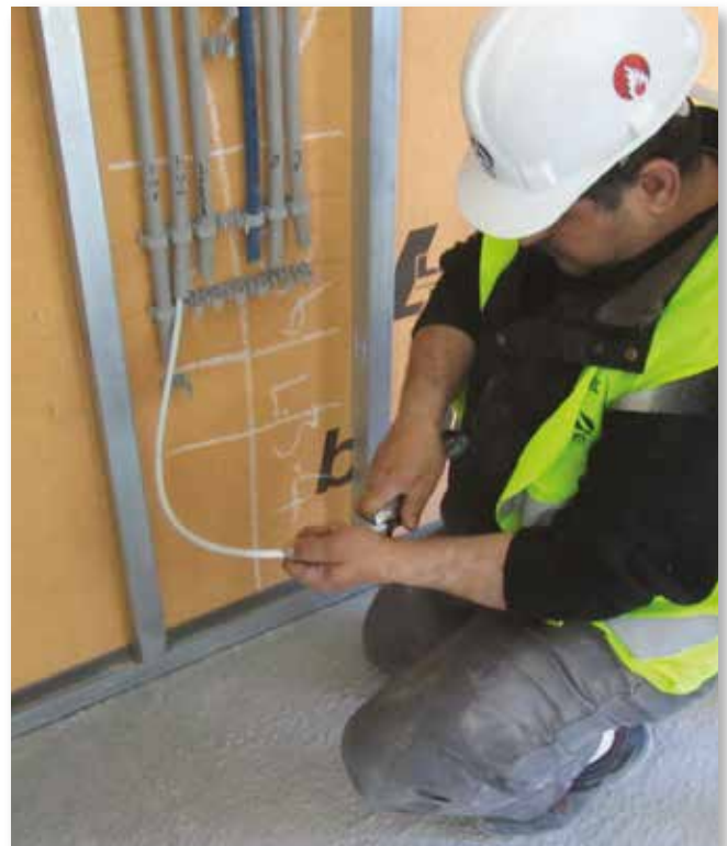
Easy stripping of cables saves time during installation.
