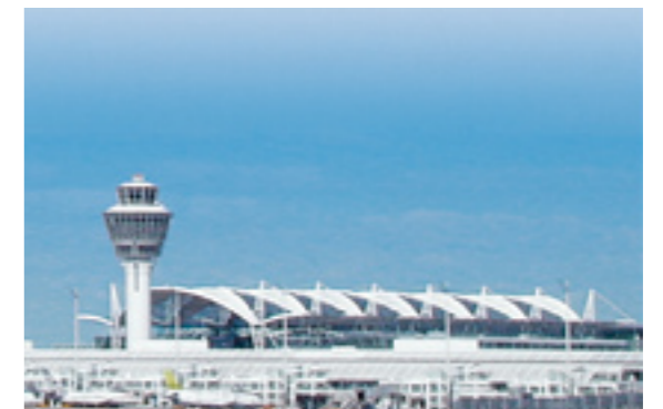
More than 100,000 OSRAM ECGs for fluorescent lamps are in use at Munich airport. They were chosen mainly for a 10 K lower tc temperature in typical luminaires. For users, this means that the ECGs last twice as long.
